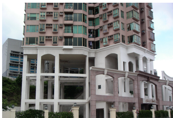
Figure 1. Combined structural system with transfer plate
