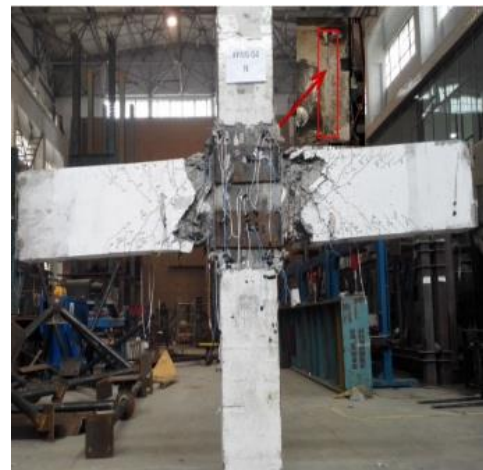
(b) Experimental failure in the nodal core area (The photograph was taken by the authors in Xian, China, on June 20, 2016) Fig. 2 Comparison of failure in the nodal core area
