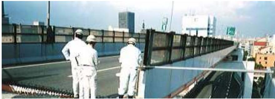
Fig. 4 Relative displacement of girder in transverse direction (about 3.5 m).
