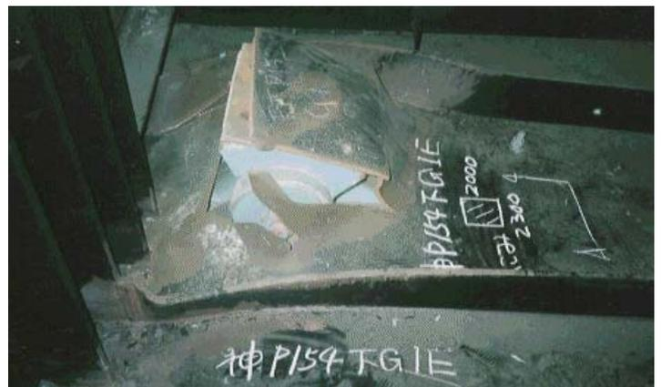
Fig. 1 Penetration of a bearing support into bottom flange.
