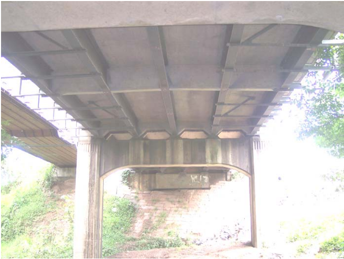
Figure 6. Underside of Redbank Creek bridge
