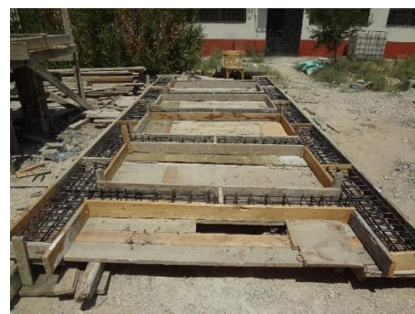
Fig. 3 Beam-column joints molds
