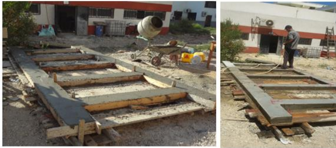
Fig. 4 Concrete specimens casting and moistening
