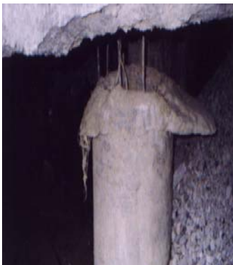
c. Pile head released from pile cap
