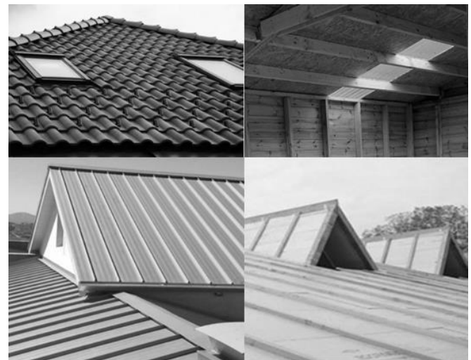
Fig. 1 Types of roofing materials; clay tiles, timber, aluminium sheets, expanded polystyrene sheets
