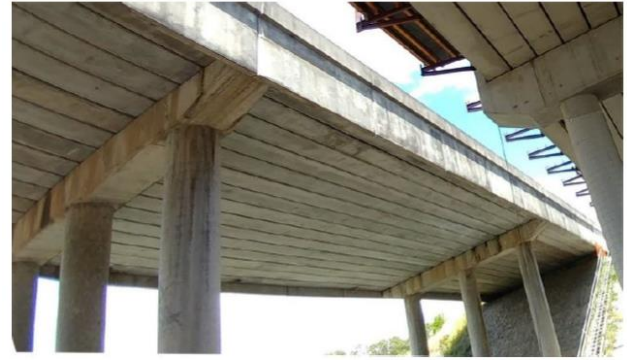
Figure 8: View of the tested bridge underneath
