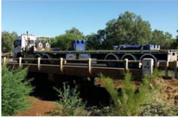
Figure 7: Load testing on deck unit bridge in QLD
