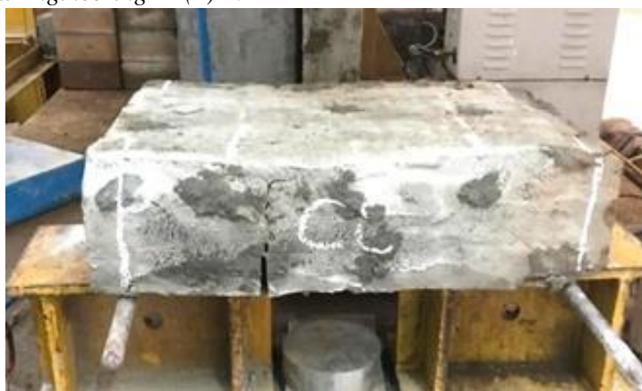
Figure 11 Failure of block masonry in flexure
