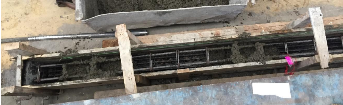
Figure 3 - wooden mold of beam.
