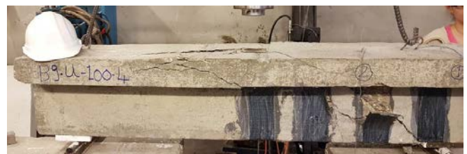
e) CFRP sheets strengthened beam B9-UW-100-4 (Set 9)
