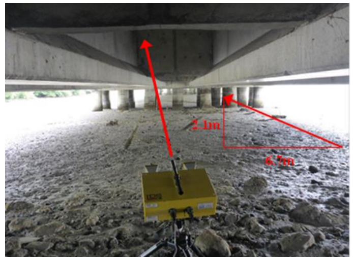
Figure 6. Testing set up of IBIS-S in trestle bridge at Terminal Teluk Lamong
