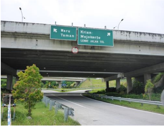
Figure 7. View of the Waru I bridge
