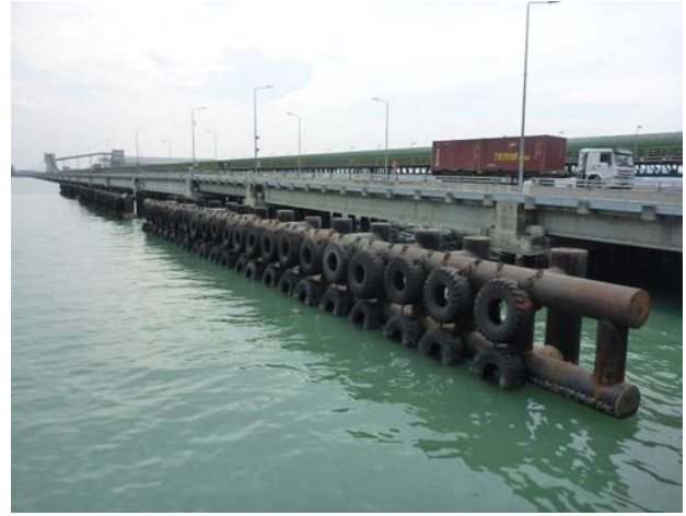
Figure 5 View of trestle bridge at Terminal Teluk Lamong
