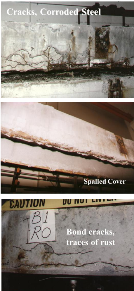
Fig. 2. Cross section and section elevation of an HC-Type precast bridge girder (above) and current girders state (below).
