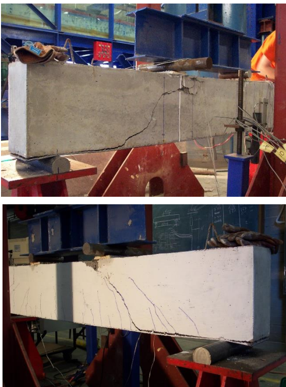
Figure 15. Failure of Beam 7 in shear acting interactively with diagonal crack-induced interfacial debonding of the CFRP.
