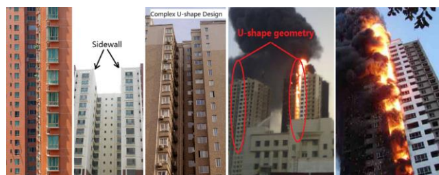
Figure 5.6. U-shaped facade wall geometry and a fire occurred in a building with U-shaped facade, Shanghai, China, 2010 (Yan et al. 2017)
