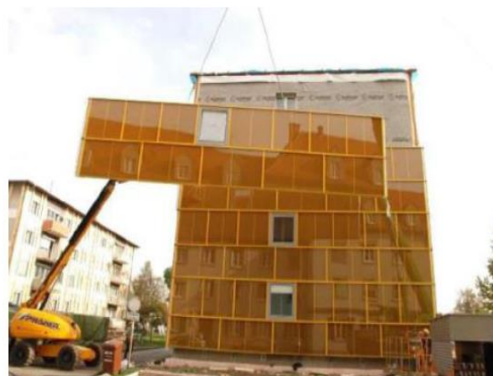
Figure 5.1 A prefabricated timber facade used in building renovation (Malacarne et al. 2016)
