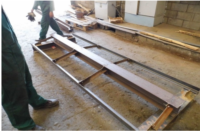
Figure 6. Angles L50×5 used to brace the compression flange against lateral buckling.
