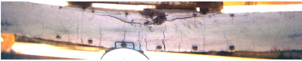
Figure 5. Failure pattern of reference beam (S0 L0).
