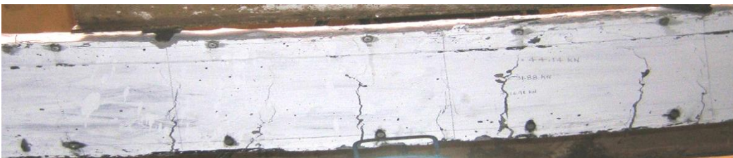
Figure 7. Failure pattern of SFRC beam (S1 L0).
