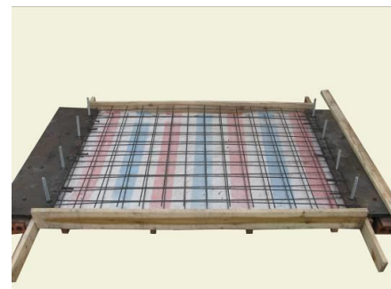
(a) Reinforcement detailing
