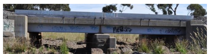
(b) Bridge, looking north.
