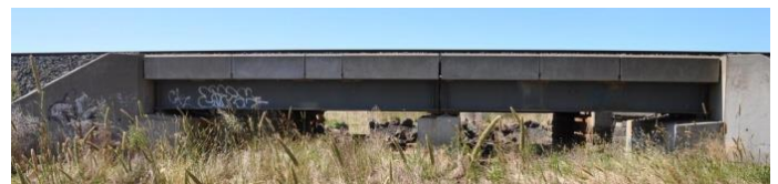
(a) Bridge, looking south.
