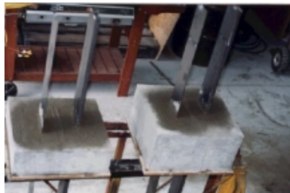
(b) Voids grouted horizontally
