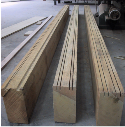
Figure 3. Timber beam strengthened with GFRP rods
